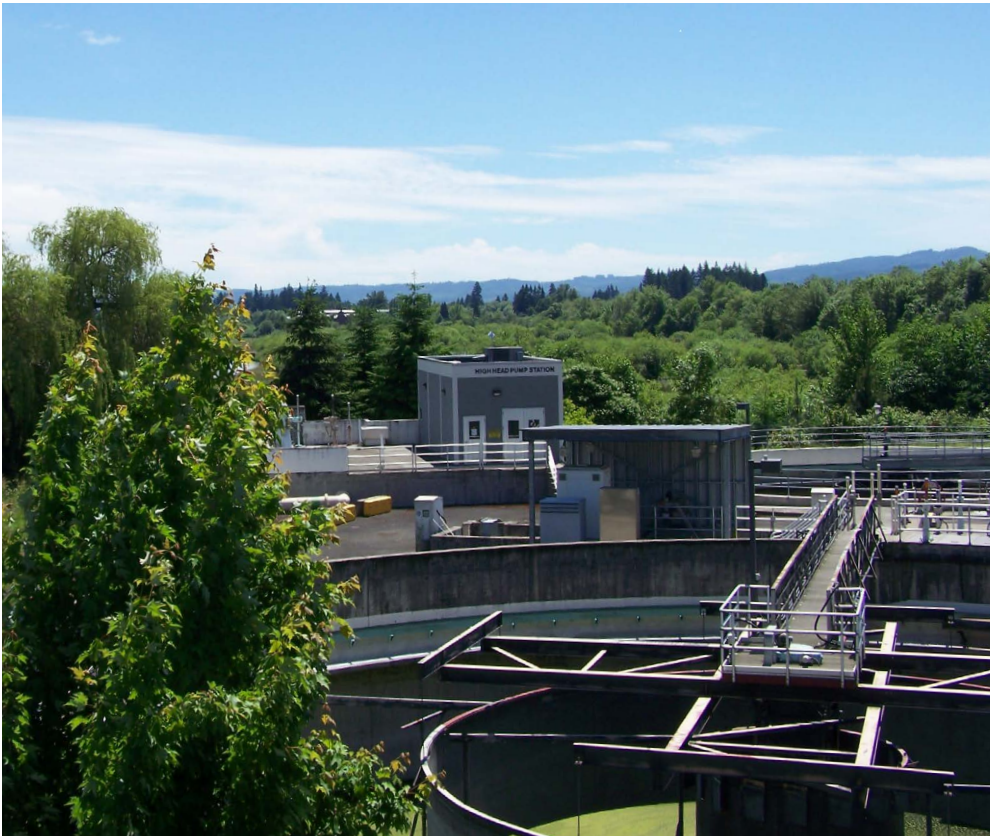
VIEW OF HILLSBORO WATER RESOURCE RECOVERY FACILITY CLARIFIERS
